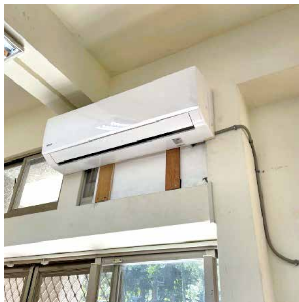
冷氣室內機裝設情況
